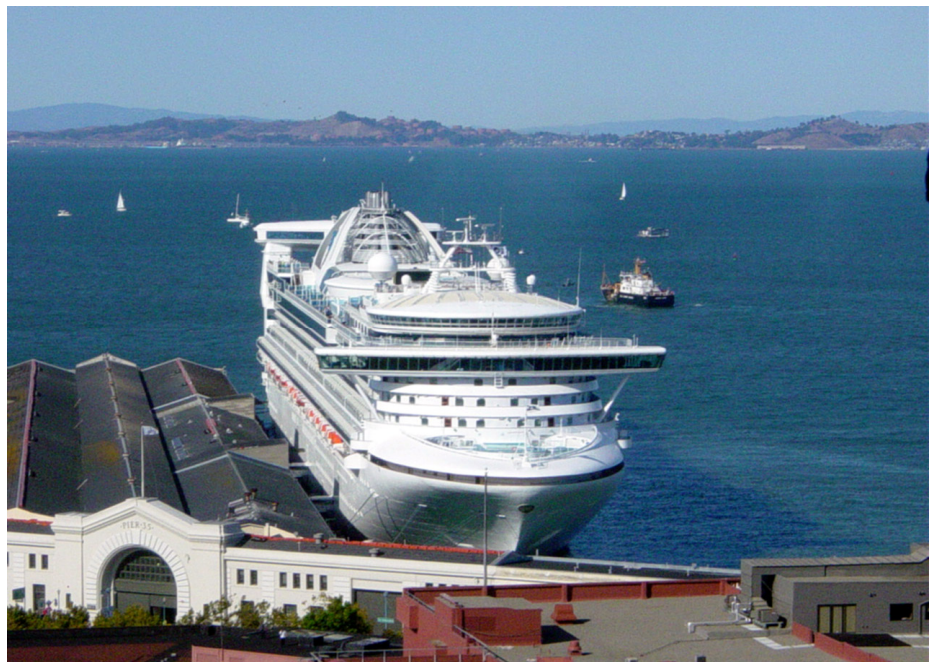
SOON TO BE IMPROVED —Pier 35, the Port's current makeshift Cruise Terminal, would receive some long-neglected repairs, while bond funds would be used to reconstruct Pier 27, which would be the home of a new Cruise Terminal.
