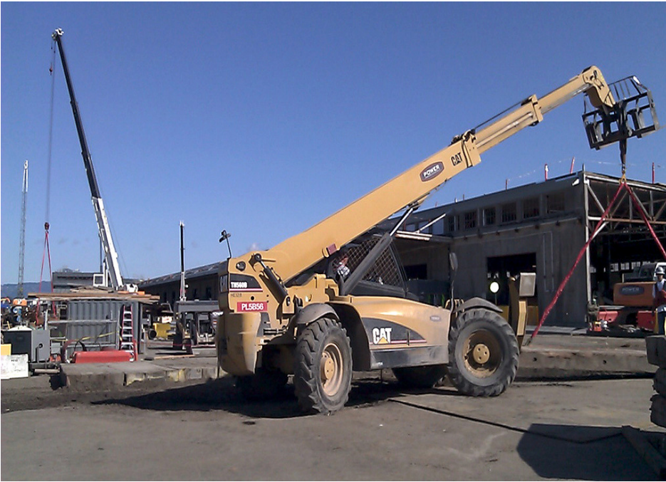
MASSIVE CONSTRUCTION —The future site of The Exploratorium is taking shape at Piers 15-17. This new jewel of our waterfront is still scheduled to open in the Spring of 2013.
