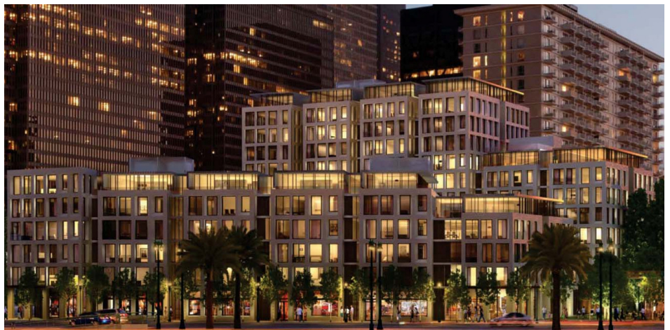
8 WASHINGTON’S HEIGHT ISSUE —Allowing this controversial project to exceed the 84-foot height limit for the development parcel opened the door for 8 Washington foes to let voters decide the issue as a referendum, the first in nearly 50 years.
