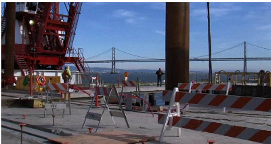
**EXPLORATORIUM PROGRESS**—Construction at the Exploratorium's new home on the Embarcadero is moving forward. The existing non-historic connector building on the east end of Piers 15 and 17 was demolished, revealing for the first time in 55 years a view out to the Bay. Recently, large 72" piles were driven 160 feet into the sea floor. In early March, the steel casings were filled with concrete.
